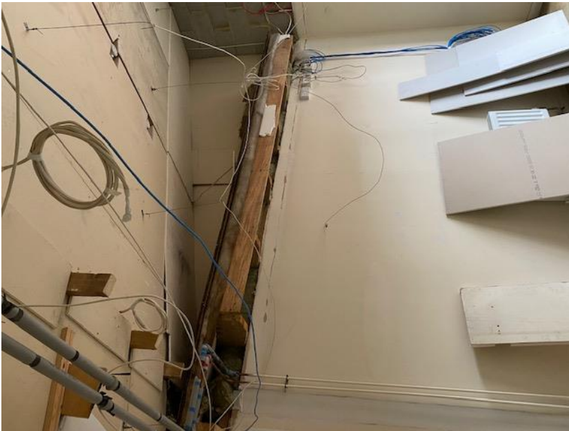
Evidence of old roof within the office ceiling void:
